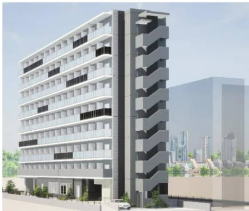
Exterior of the building / 外観
